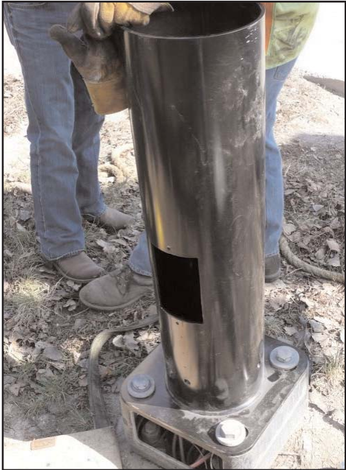
Duratel pole base designed for installation on legacy footings
